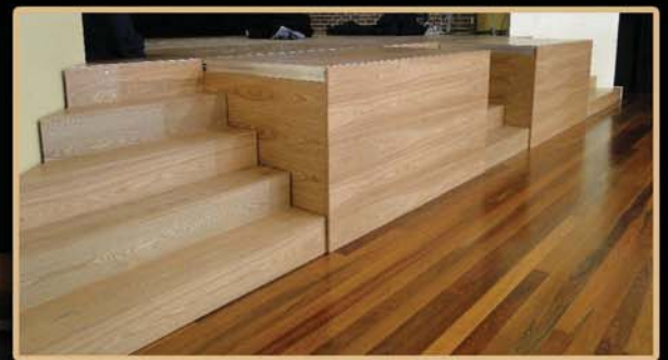
Permanent stage refurbishment with QUATTRO
